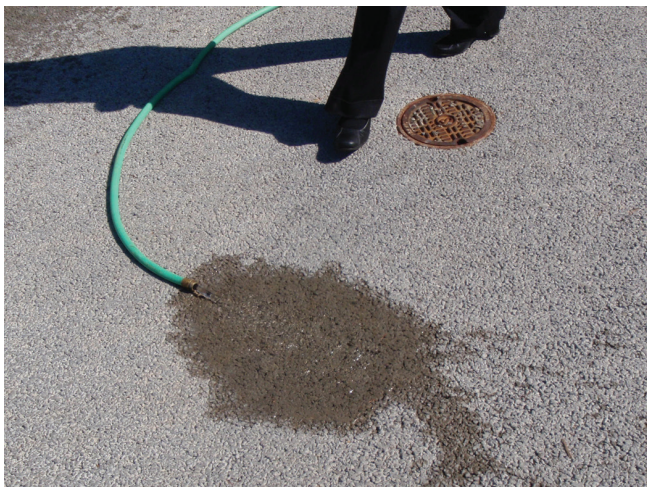
Figure 1. Typical permeable pavement.
