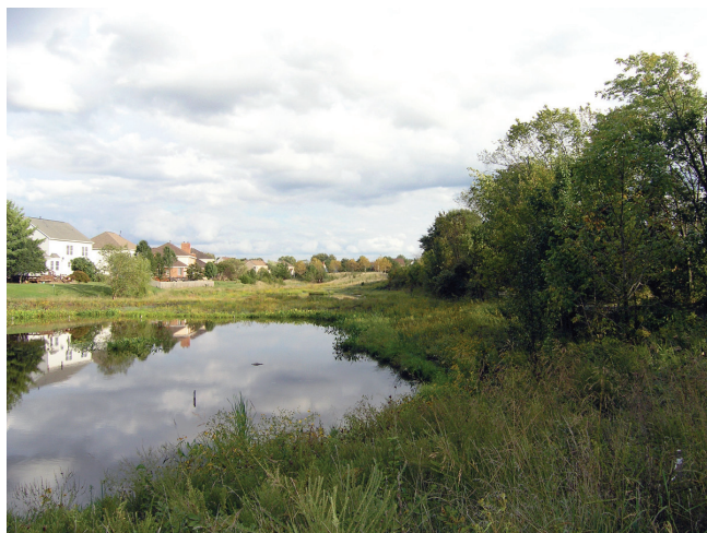
Figure 1. Typical wet pond (VA-DCR 2011).
