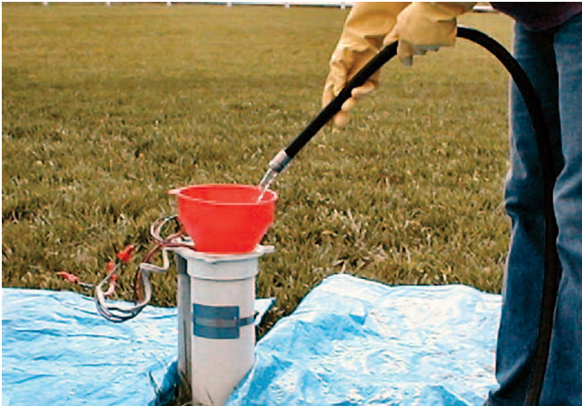
Figure 2. Circulate water in the well and wash down the inside of the casing. Source: Minnesota Department of Health. www.health.state.mn.us/divs/eh/wells/waterquality/disinfection.pdf .
