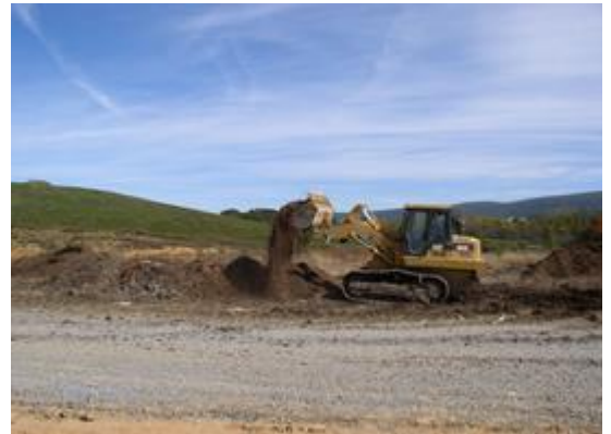
Composting Mortality at the Shenandoah County Landfill
