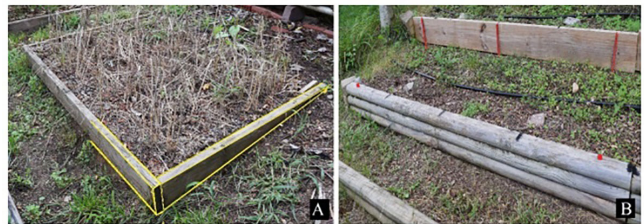
Figure 2. A) A three-sided 6-by-4-foot raised bed made from 8-inch untreated boards with sideboards (yellow outline) tapered to fit the topography. B) Two bed sections framed on the downhill side only using stacked landscape timbers (lower section) and a single 2-inch by 8-inch by 10-foot treated board (upper section). The timbers are secured with rebar (red) driven through 5/8-inch holes while the board is pinned in place between the rebar (red) and backfilled growing media.
