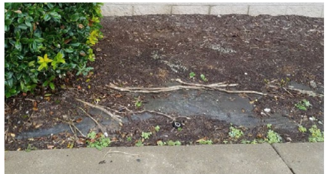
Figure 2. The landscape fabric covering this garden area has become clogged over time, not allowing water through and forcing the shrub's roots to grow upwards to the surface to gain access to oxygen and moisture.
